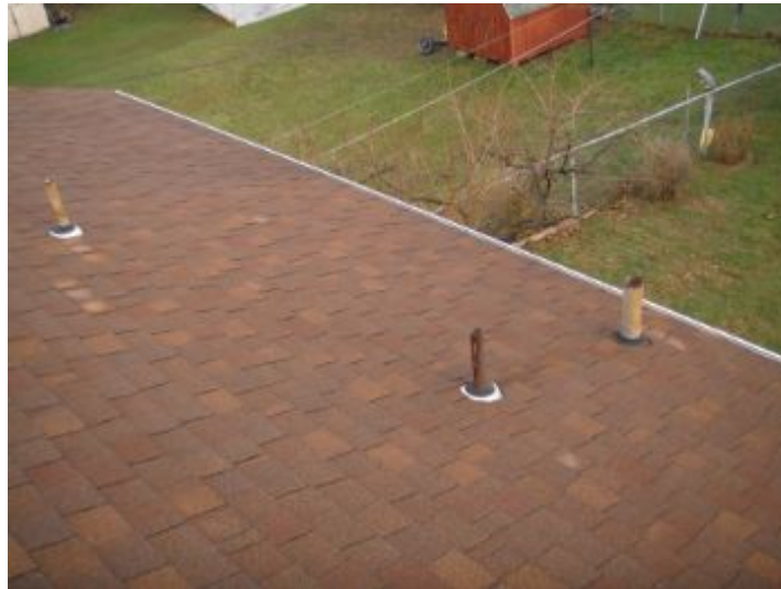
Penetrations/flashings appeared in good condition, at time of inspection.
