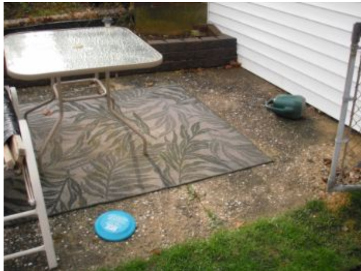
Rear concrete patio appeared in good condition.
