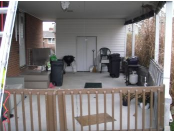
All components of carport in very good condition with recent upgrades.
