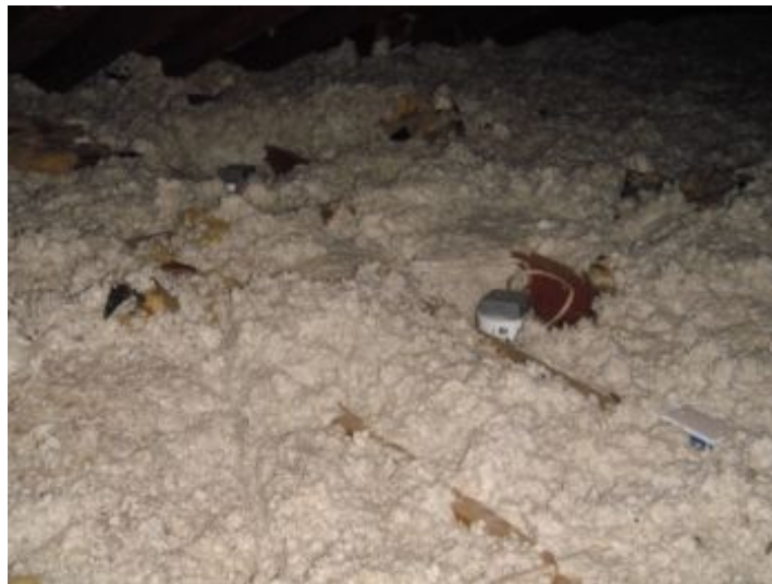
Insulation appears adequate.
