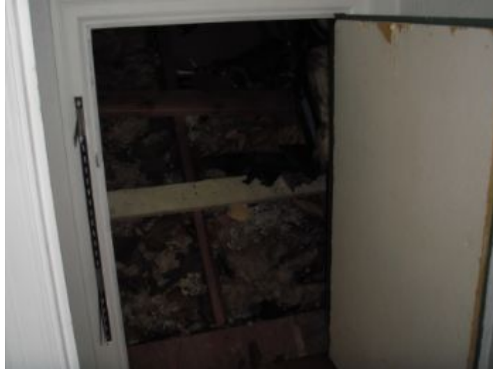
Attic access in Living Room closet.
