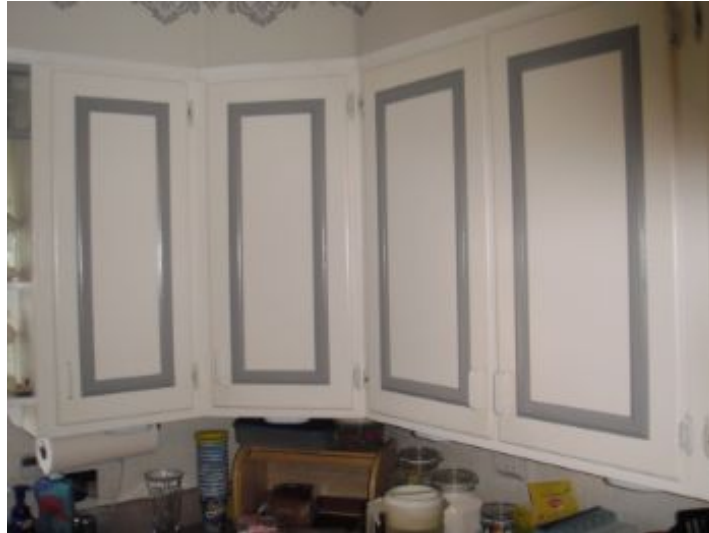
Well maintained Kitchen cabinets
