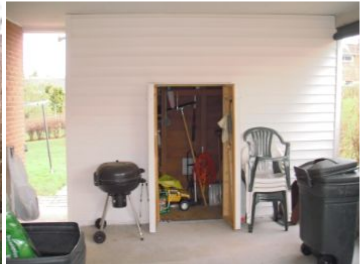
Carport storage room.
