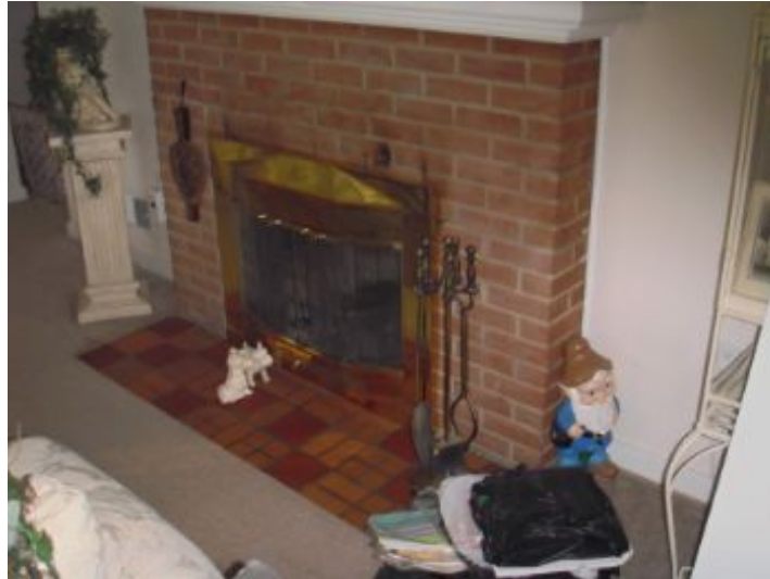
Wood burning fireplace in Living Room.
