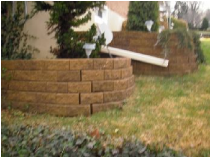
Retaining walls in good condition.
