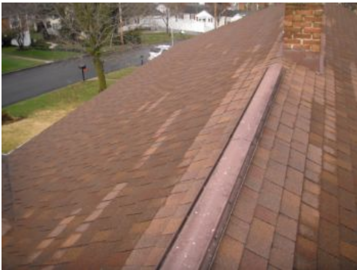
Roof covering appeared in good condition.
